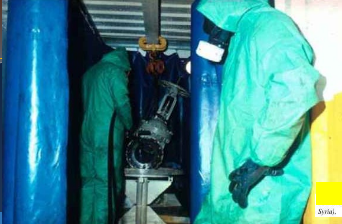
Workers wearing personal protective equipment decontaminating a valve inside an on-site facility (courtesy: National Radiological Protection Board, UK).
